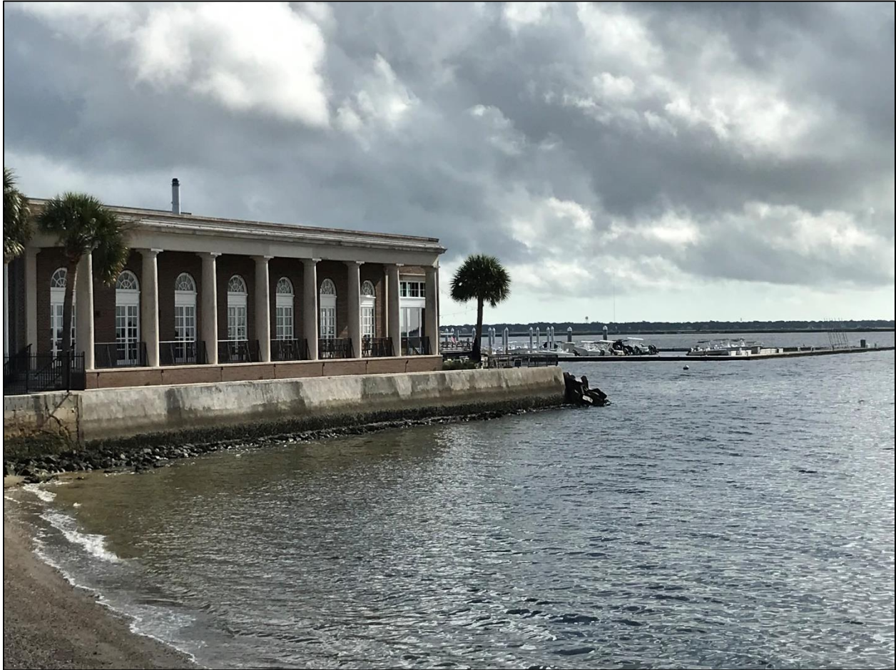
Figure 4-11. Seawall by the Carolina Yacht Club along the Charleston Harbor. It is reinforced at the toe with rip rap, which continues around the corner along the east side of the yacht club (out of view in this photo).
