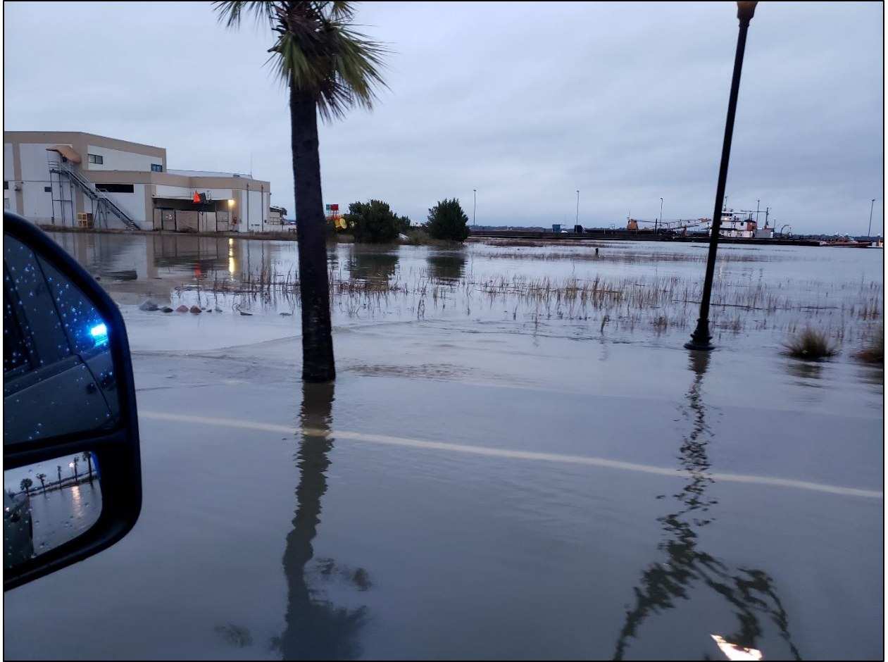
Figure 4-28. Inundation on Lockwood Blvd/Broad Street and the perimeter saltmarsh by the U.S. Coast Guard station at high tide during a storm in December 2019.
