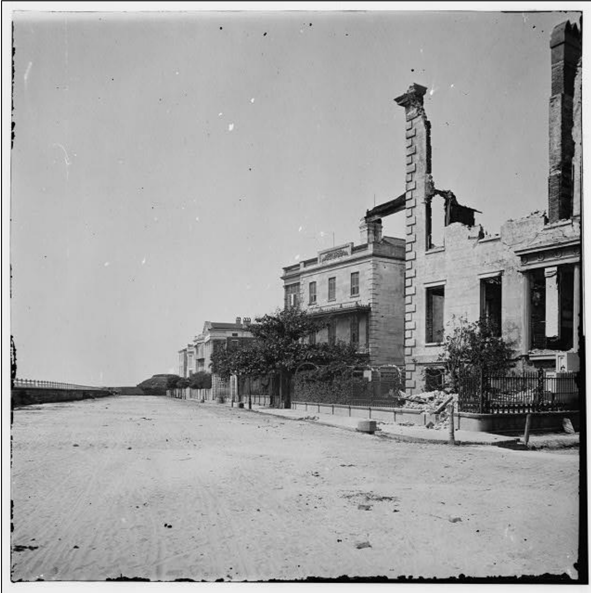
Figure 4-14. “Charleston, S.C. Houses on the Battery damaged by shell-fire.” Photographed by George N. Barnard, 1865.
